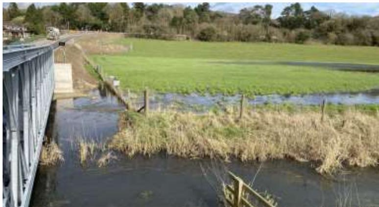
River water spilling into the floodplain through a damaged section of the bank of the R. Misbourne at Bottom House Farm Lane (c) Allen Beechey
